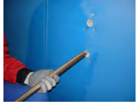
Epoxy cartridge filling is performed
