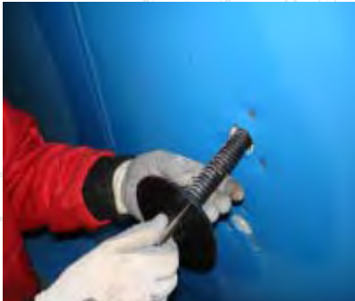
„Screwing“ in the anchor outside threading
