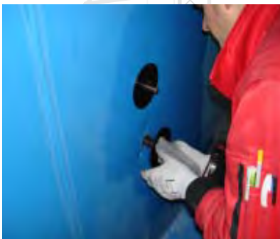
Placement of second anchor
