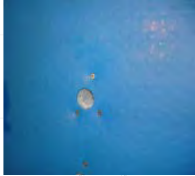
Drill hole prepared for filling with epoxy cartridge
