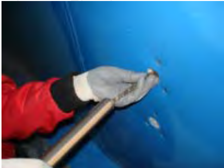
Filling of Sikadur 31
